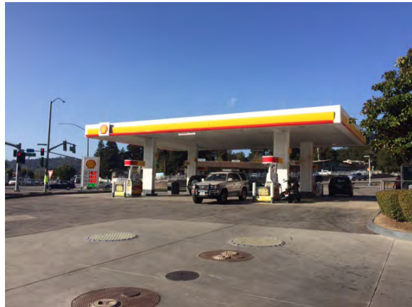
Shell Gas Station
